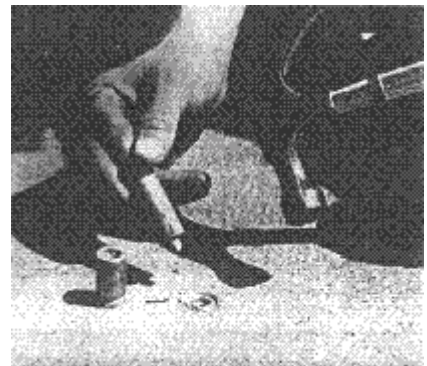
Fig. 4. Installing the lead anchor. The flared end goes down.
