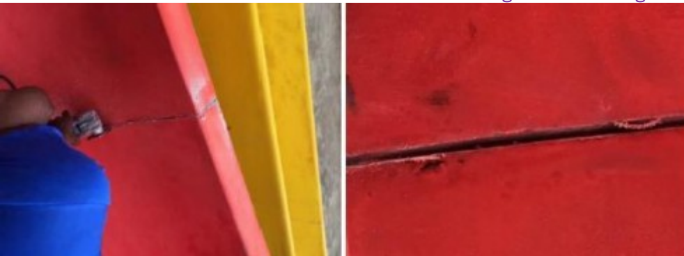
Figure 7: Removing Old Filler
