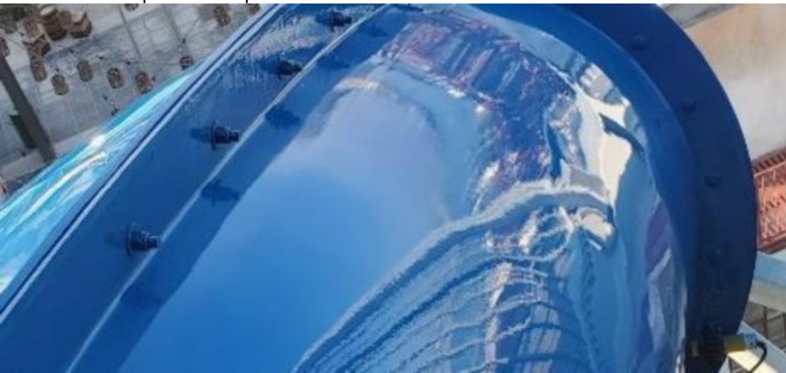
Figure 73: Inspect Finished FRP for Drips or Runs
