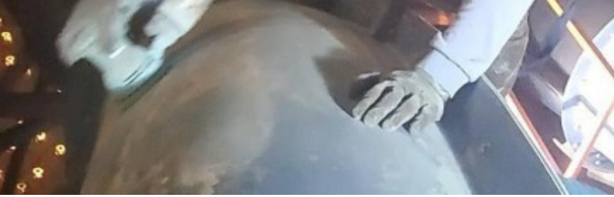
Figure 70: Sanding FRP for Clear Coat
