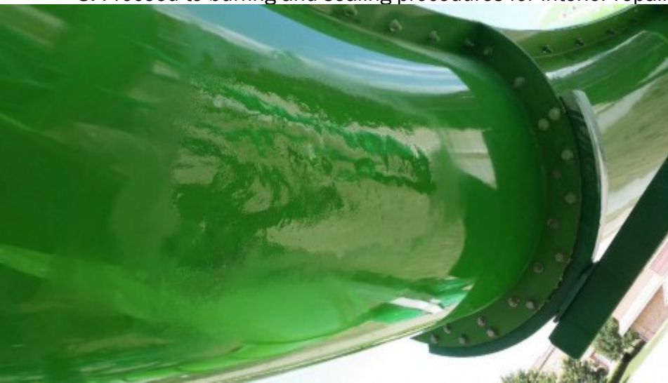
Figure 56: Gelcoated Large Repair, Outside
