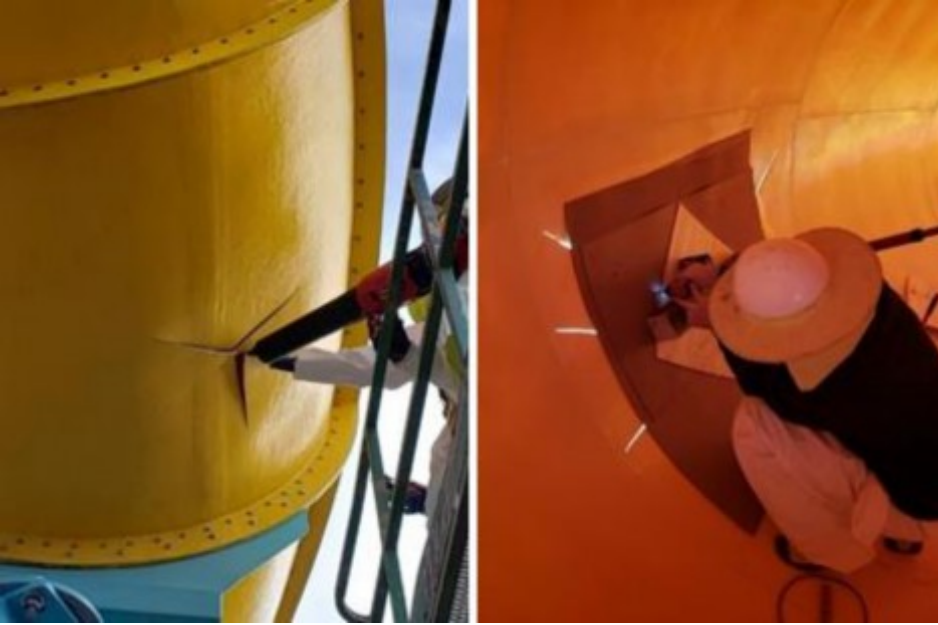
Figure 62: FRP Deformation Repair Preparation
