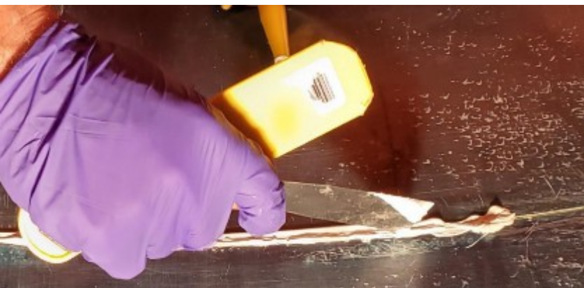
Figure 11: Pack in Joint Filler
