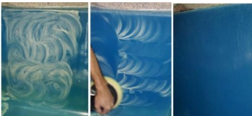
Figure 6: Buffing and Waxing Shutdown Lane FRP
