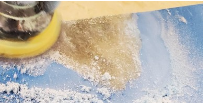
Figure 40: Sanding Fiberglass Repair
