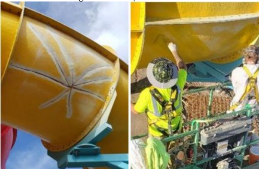
Figure 63: FRP Deformation Repair Grinding and Fiberglass Application
