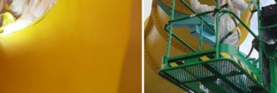
Figure 64: FRP Deformation Repair Gelcoat and Clear Coat Finishing
