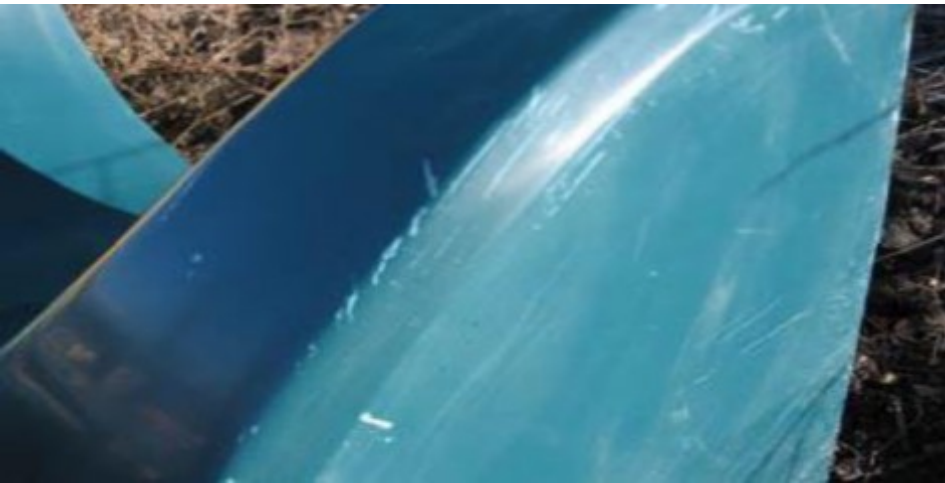
Figure 22: Scratches in Gelcoat
