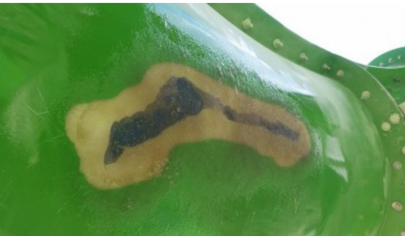
Figure 39: Cured Fiberglass Repair, Outside
